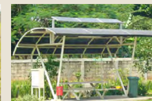
Solar power system installed on plant grounds
