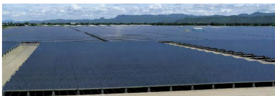
73 MW mega solar plant, one of the largest in the world (Lop Buri Province, Thailand)
