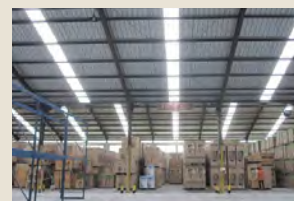
Roofing that lets in natural light
