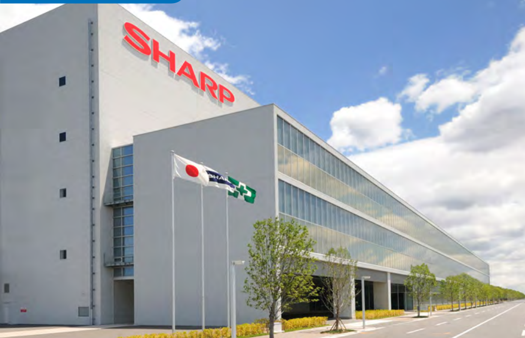
Solar cell plant at GREEN FRONT SAKAI (operations began March 2010)
